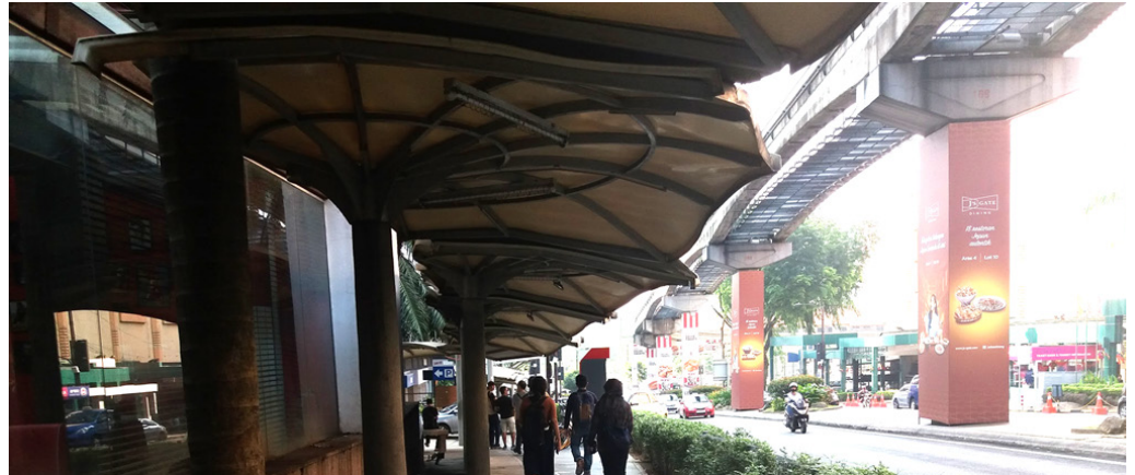
Connecting canopy along the sidewalk
