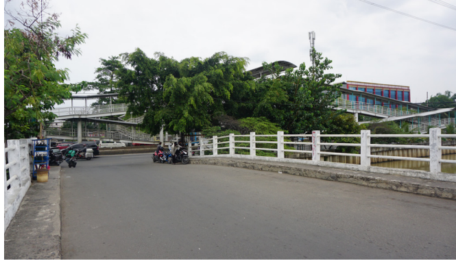
Location 1 Existing condition
