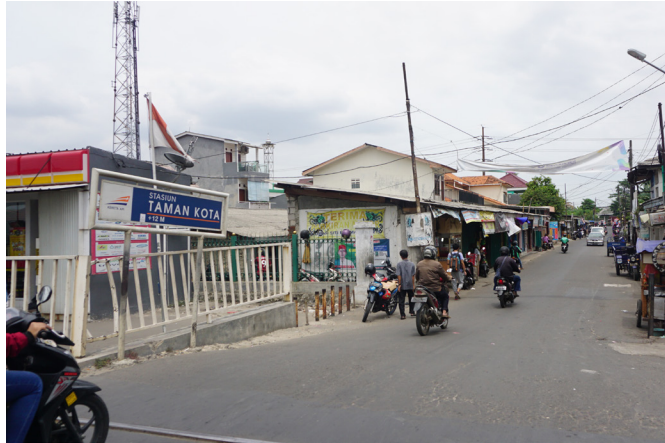
Location 2 Existing condition
