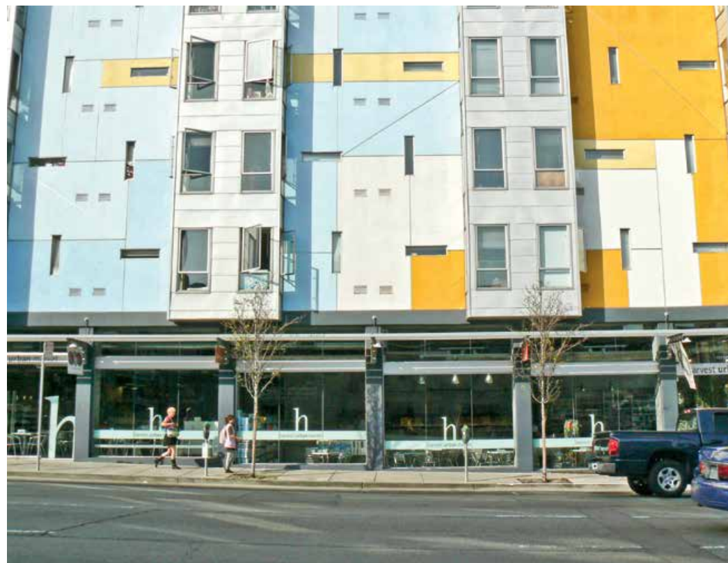
This development in the Soma district of San Francisco, California, USA, includes affordable housing and commercial uses with active frontage.
