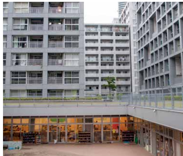
This ground floor kindergarten facility at Shinanome, Tokyo, Japan, is conveniently accessible to the parents and children living above and around.
