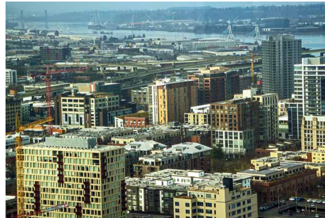
The redevelopment of a former industrial site in the Pearl District of Portland, Oregon, USA, combines high densities in work and residential uses integrated with great walkability and sustainable transportation options.
