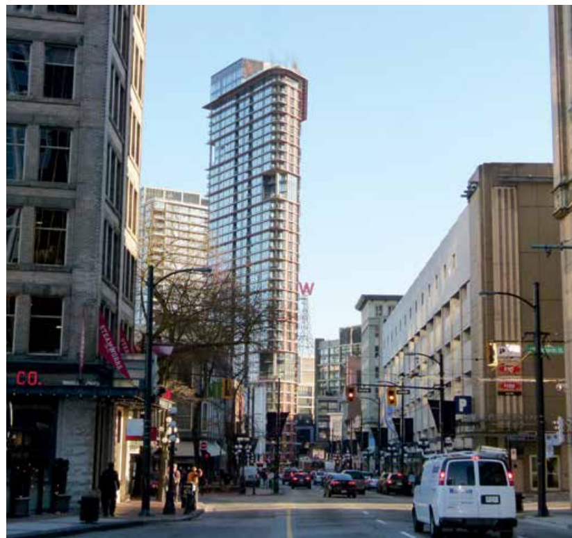
This mixed use development in Gastown, Vancouver, Canada, adds infill density to neighborhood well served by transit and integrates market rate and affordable housing with commercial, offices, and education activities.
