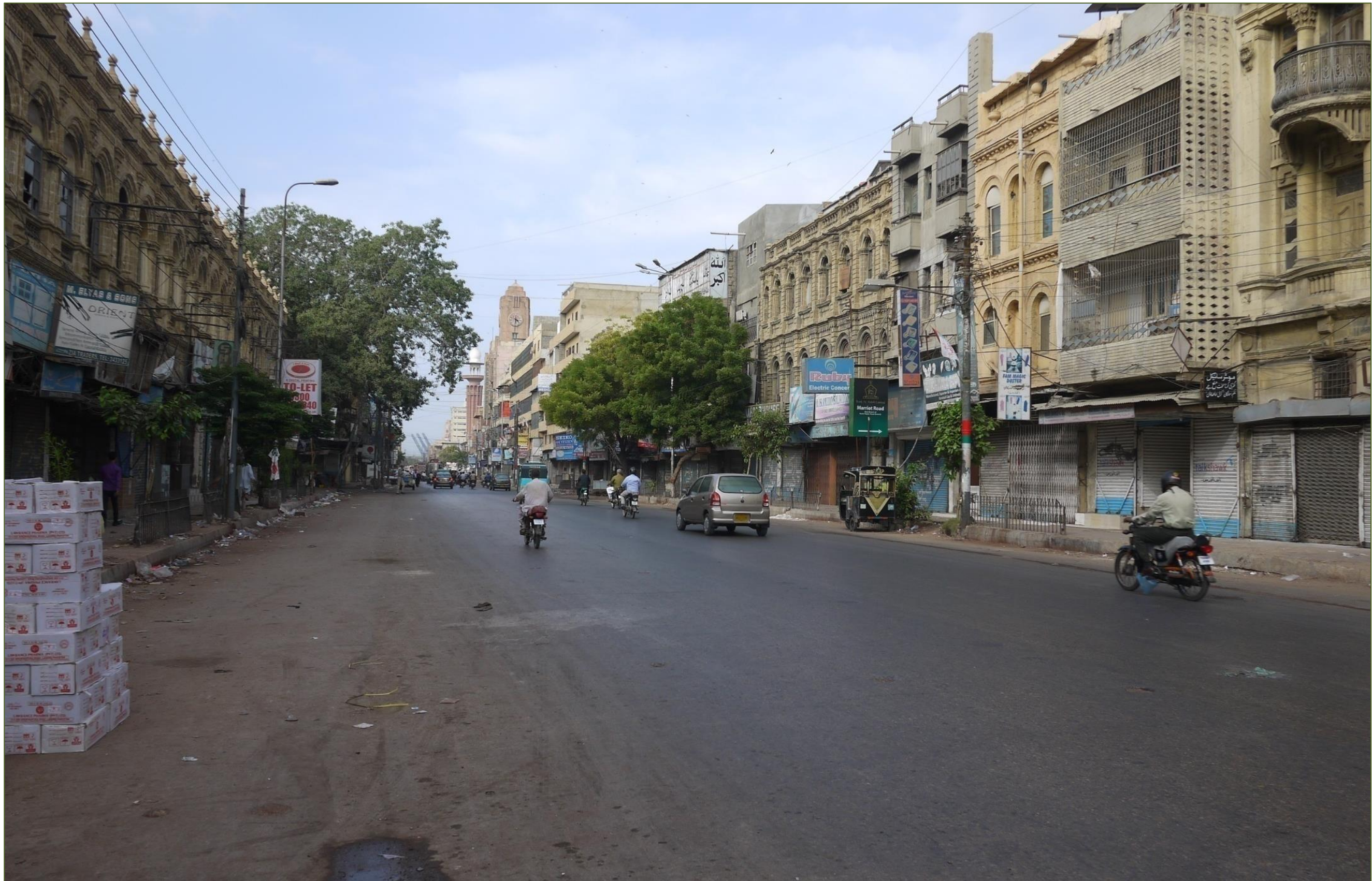
Figure 5.19 Denso Hall Existing
