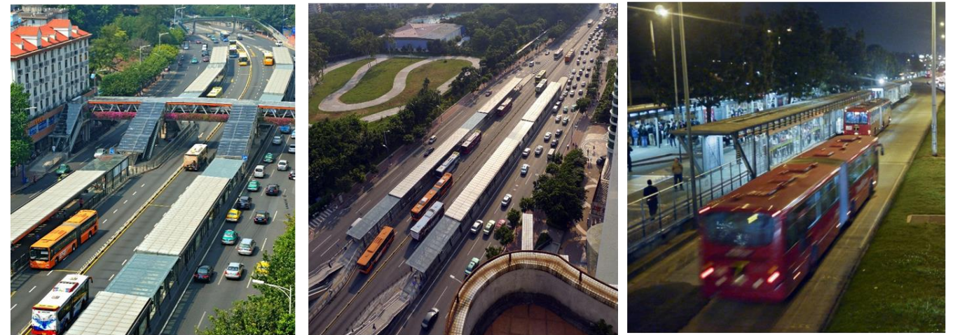
Application of Sub-stop in Guangzhou BRT
