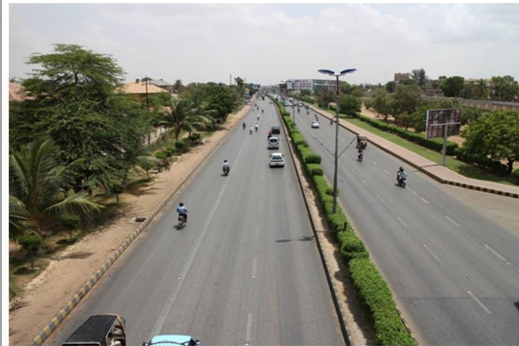
Mid Section of Sharah-E-Faisal Road near Military Base Area
