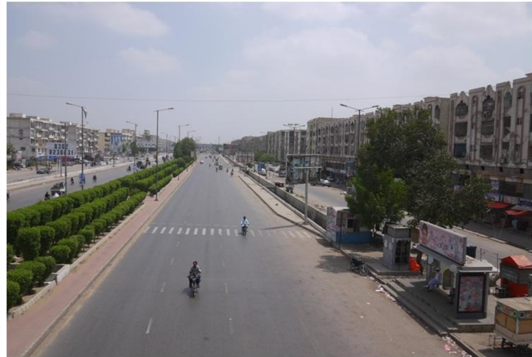
North Part of Green line on Shahrah e Shershah Suri Road (84.2meter)
