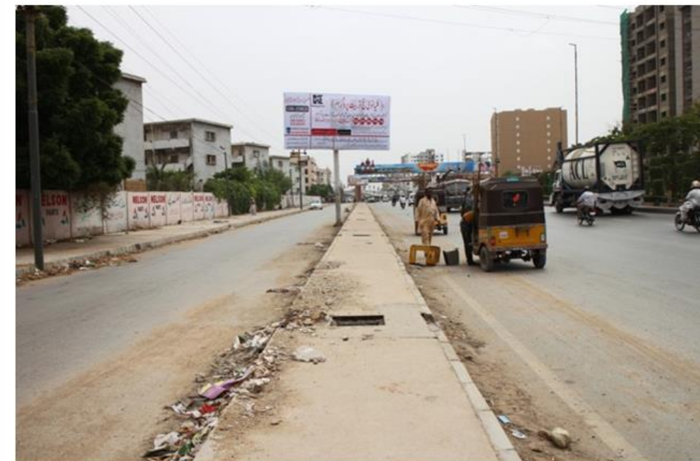
Mid Section of Brown line with on-going development
