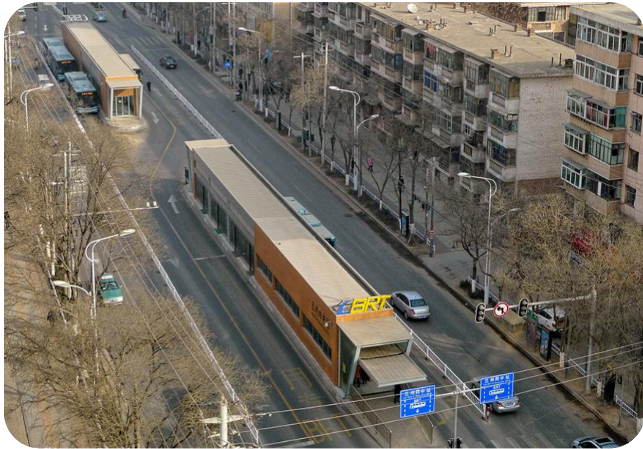
Figure 5. 12 Example of Split Station in Chinese BRT systems in Lanzhou (left) and Yichang (right)
