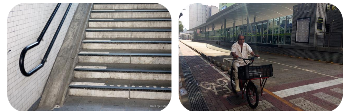
Figure 5. 39 Bicycle Guiding Rail (left) and Cycle Lane next to BRT Corridor (right).
