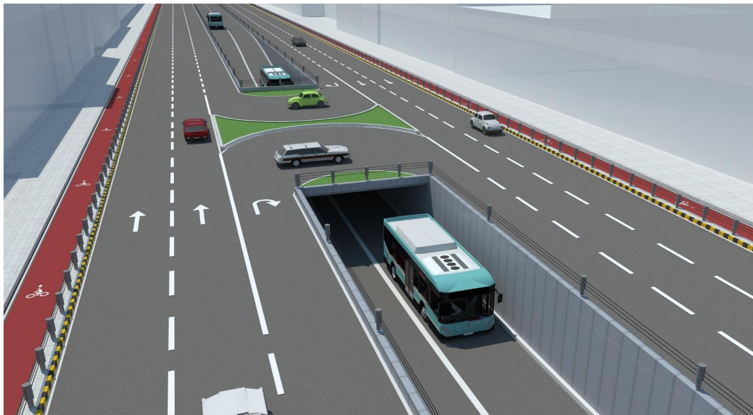
Figure 8. 3 BRT-only Tunnel to avoid U-Turn Movement for general traffic.
