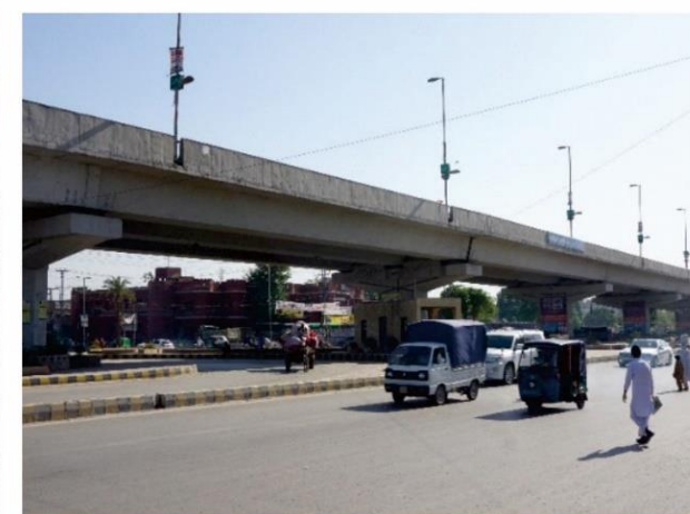
Grand Trunk Rd Looking west
