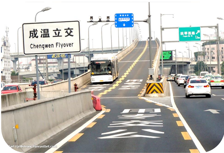
Figure 4. 8 Elevated BRT Corridor in Chengdu, China
