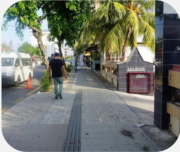
Continuous sidewalk even on driveway along Jalan Pantai Cenang
