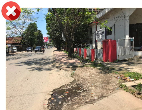
Example of pedestrian lane discontinued at driveway (top left)
