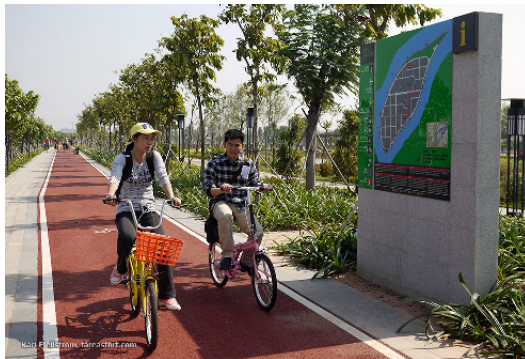
Left: Pigmented asphalt for a cycling lane in Guangzhou, China (source: Karl Fjellstorm, Far East Mobility)
