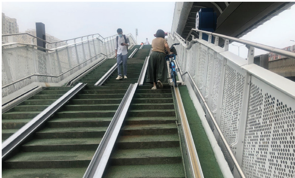
RIGHT: In Beijing, China, wheel ramps allow bicycle riders to more easily access the elevated cycle highway. SOURCE: ITDP China
