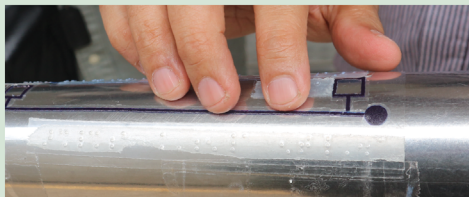
Trial of tactile and braille information on entrance handrails
