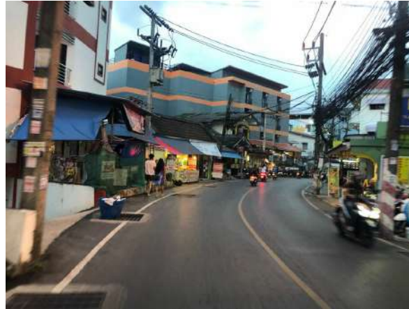
No sidewalk at main road
