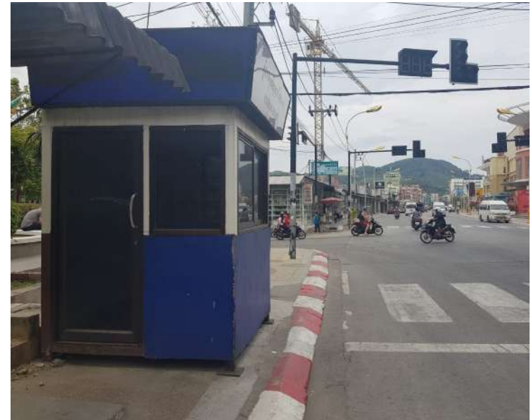
Sidewalk occupied by utilities
