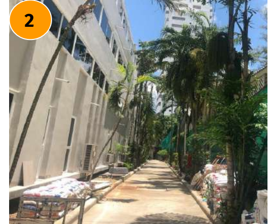
Pedestrian path blocked by wall
