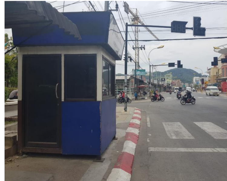
Sidewalk occupied by utilities
