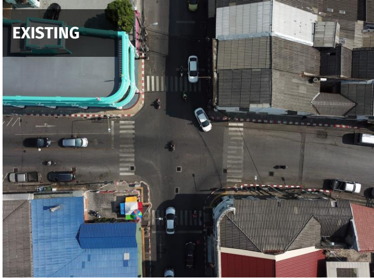
Intersection Between Dibuk Road - Yaowarat Road
