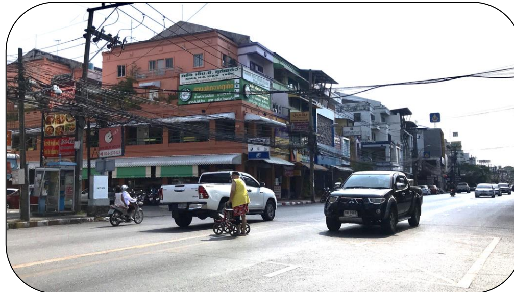
Mobility-impaired person tries to cross the road without any safe crossing facility
