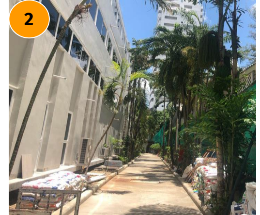
Pedestrian path blocked by wall
