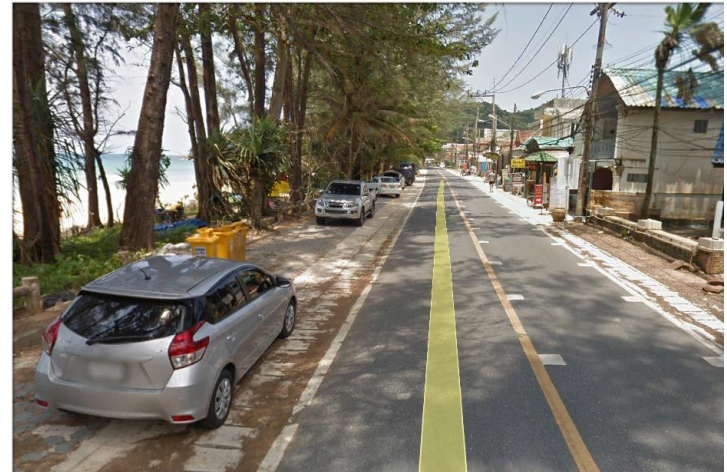
A Section - The road width on proposed new route is adequate to accommodate bus operation
