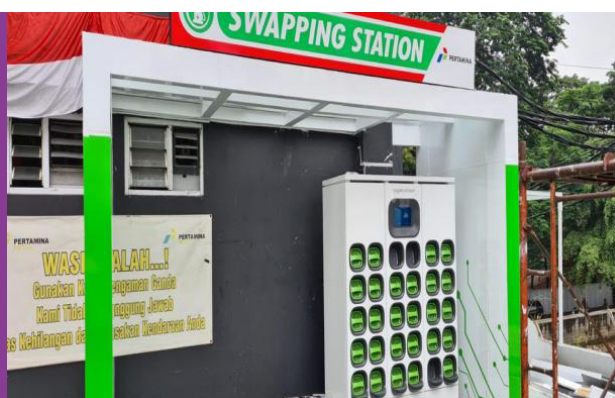
Figure 11. Battery swap station provided by Pertamina 27 (Source: Republika.co.id/Intan Pratiwi )
