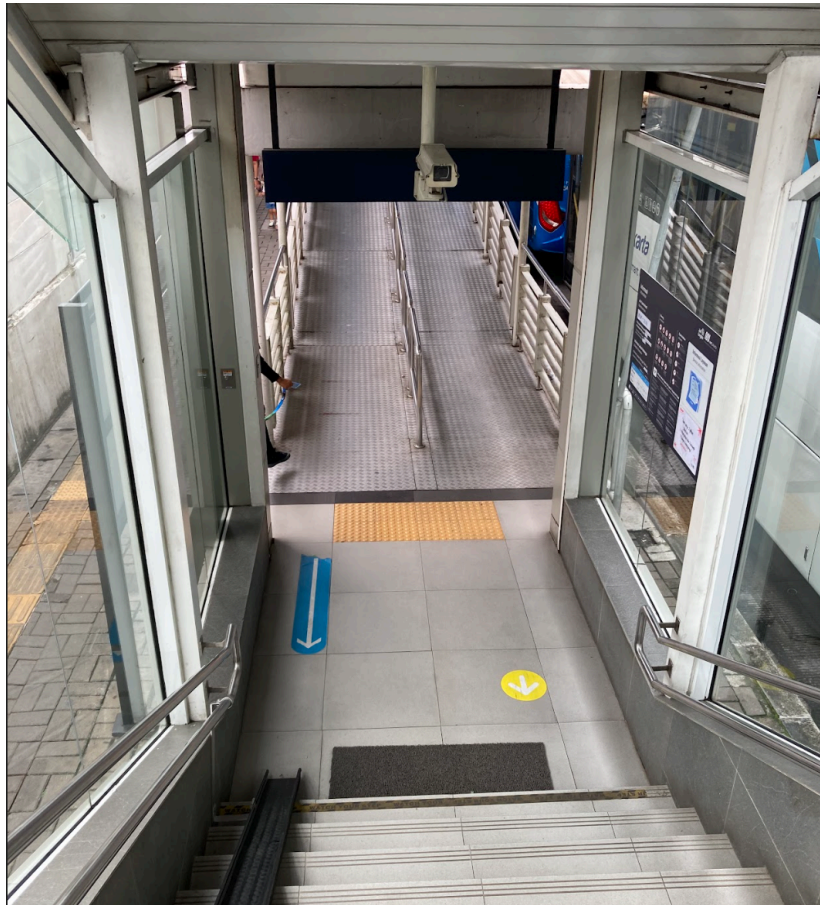
Figure 11 Lack of Wayfinding at Lebak Bulus
